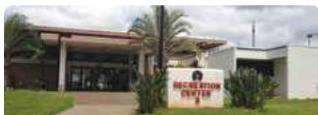
REC CENTER 3 | BUSINESS OFFICE
