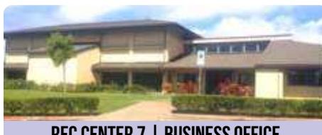
REC CENTER 7 | BUSINESS OFFICE
