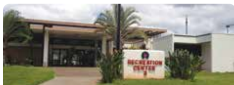
REC CENTER 3 | BUSINESS OFFICE
