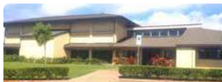
REC CENTER 7 | BUSINESS OFFICE
