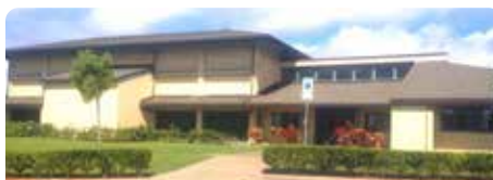
REC CENTER 7 | BUSINESS OFFICE
