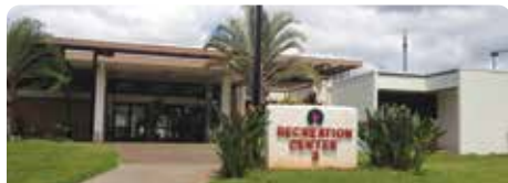
REC CENTER 3 | BUSINESS OFFICE
